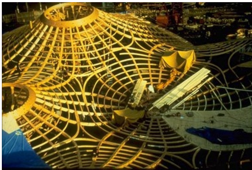
Figure 5. Bad Dürreim funicular timber grid shell under construction.
